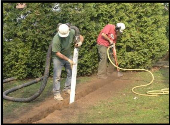
The proposed footings, along with another trench 5 metres from the gable end, were marked out by the architects and the concrete and crazy paving broken up. A 600mm deep trench was then excavated. The soil was broken up with an AirPick and removed using a soil vacuum unit. This method made it possible to retain even the smallest roots. The location and origin of root were then noted by using the proposed footings as a line transect.
