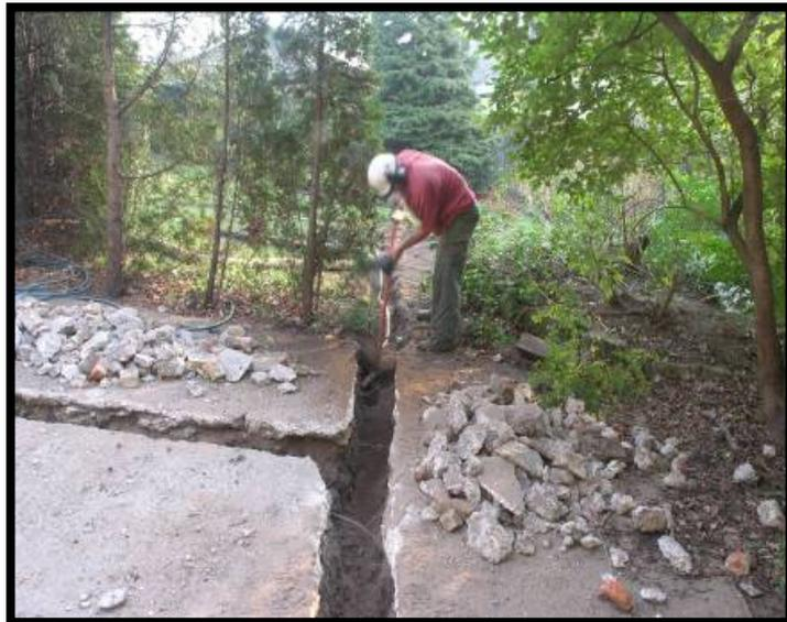
Tree roots found under the impermeable concrete, illustrated in this photograph, were clearly growing towards the area of garden that offered better rooting conditions. However, this area of garden was outside the RPA yet the roots found here could be consider as the most significant to tree health and survival.
